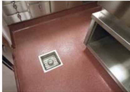
Coving prevents dirt from gathering in corners of the kitchen and makes it easier to clean. As part of the coating work, drains and channels were integrated precisely into and level with the floor.
